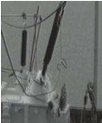
Broken bushing
