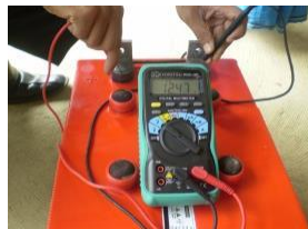
Measuring Battery Voltage
