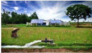
602 Solar Irrigation Pumps in Operation
