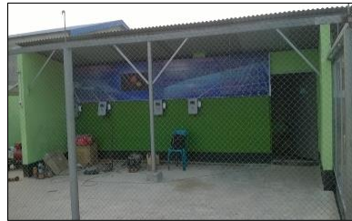
Solar charging station
