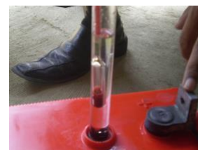
Measuring S.G of Battery
