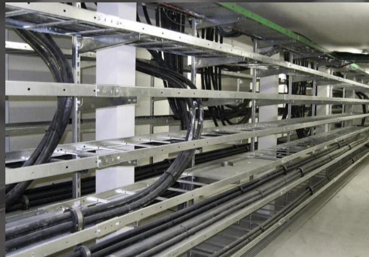
2. Underground Cable (Underground or UG)
