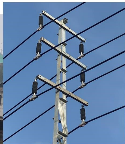
MVCC 66KV Installations
