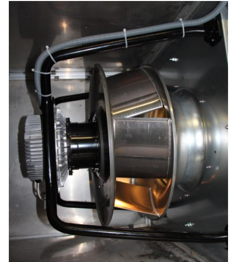
radial fan with direkt drive (motor+VFD)
