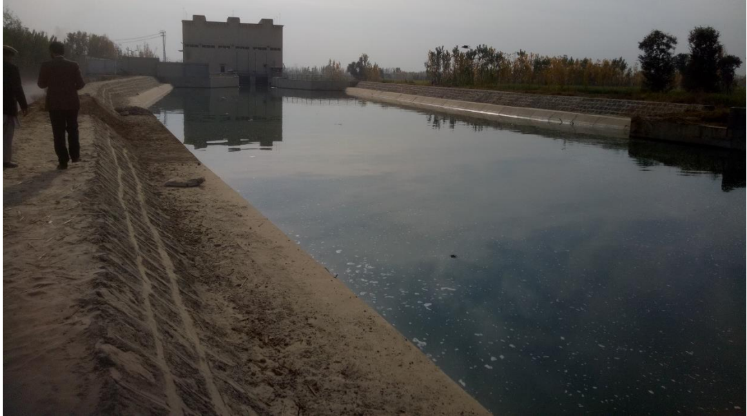
Annexure- II Fig: 1-3: Front View of the 2.6 MW Machai Hydropower Project
