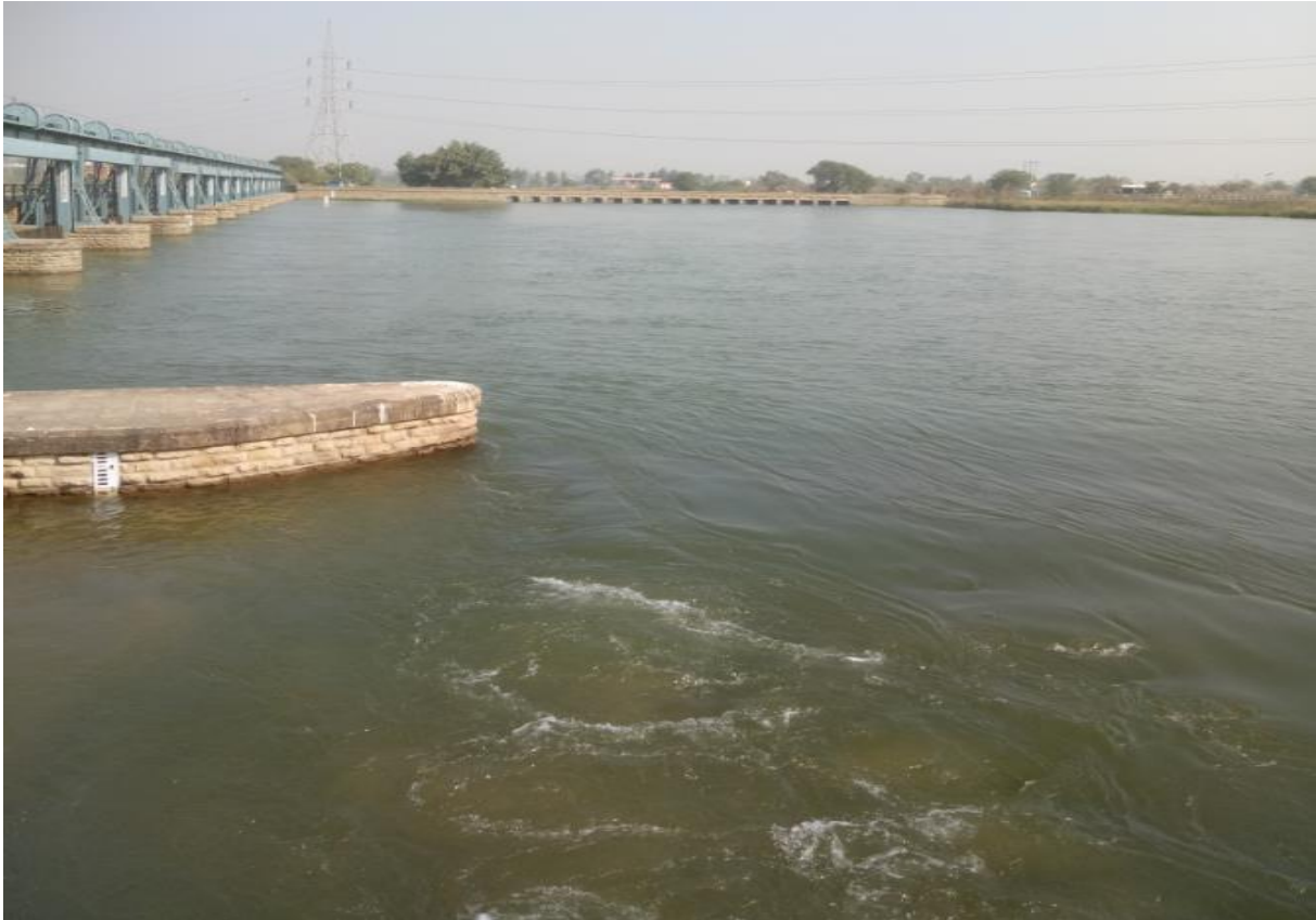
Figure 3-2: Upper Jhelum Canal at water level crossing Jaggu Head works.
