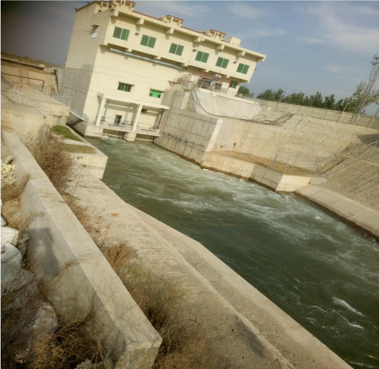
Annexure- II Fig: 0-5: Rear view of the 2.6 MW Machai Hydropower Project
