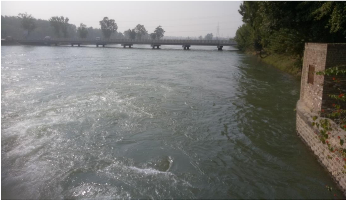
Annexure –III Fig: 0-5: Downstream of the upper Jhelum canal at Jaggu water level crossing.
