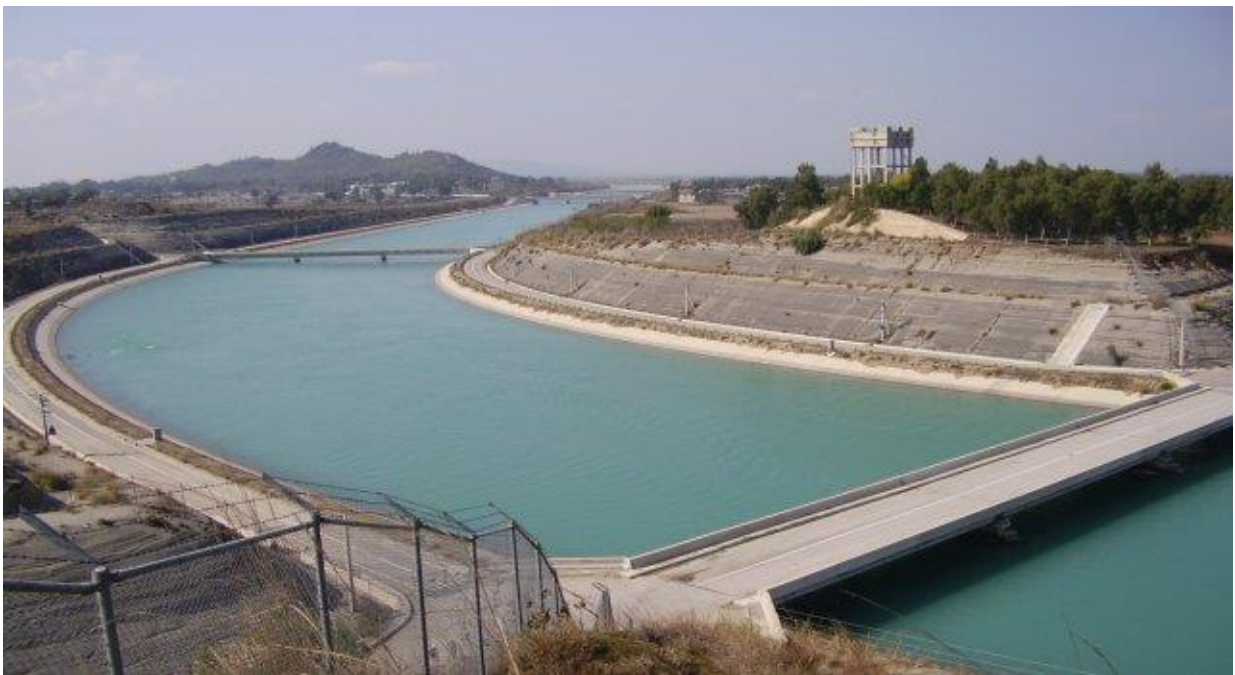
Figure 0-1: View of the Ghazi Brotha power canal originating from Ghazi Town
