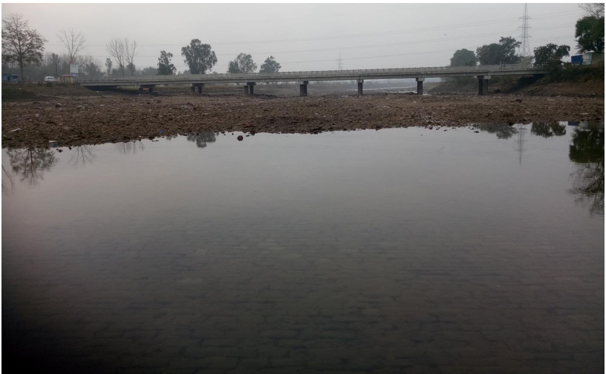
Annexure –III Fig: 0-8: Downstream of the upper Jhelum canal at Jaggu water level crossing after annual shutdown.
