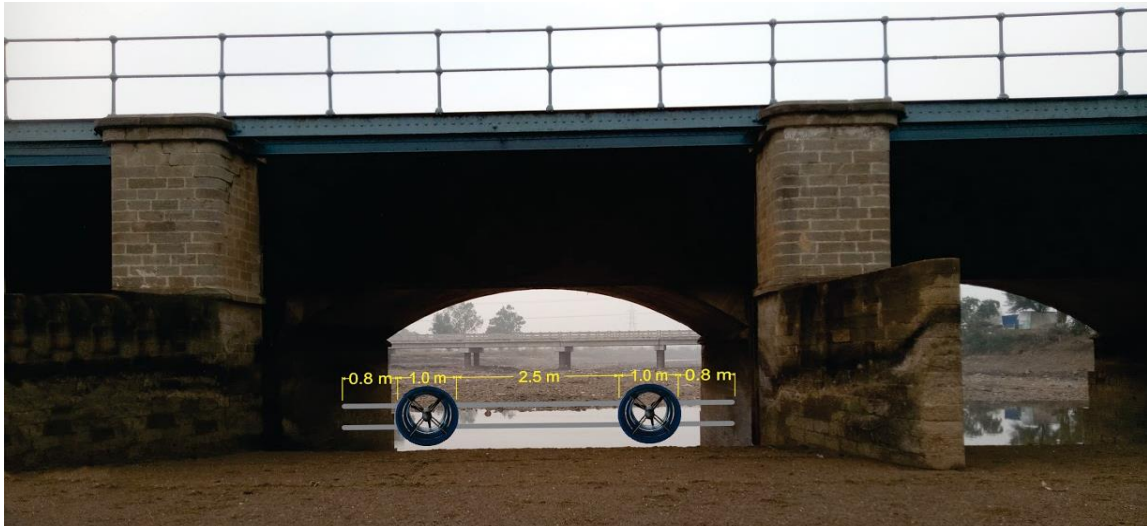
Figure 0-2: Turbine distribution with in one channel under the bridge at Jaggu level crossing
