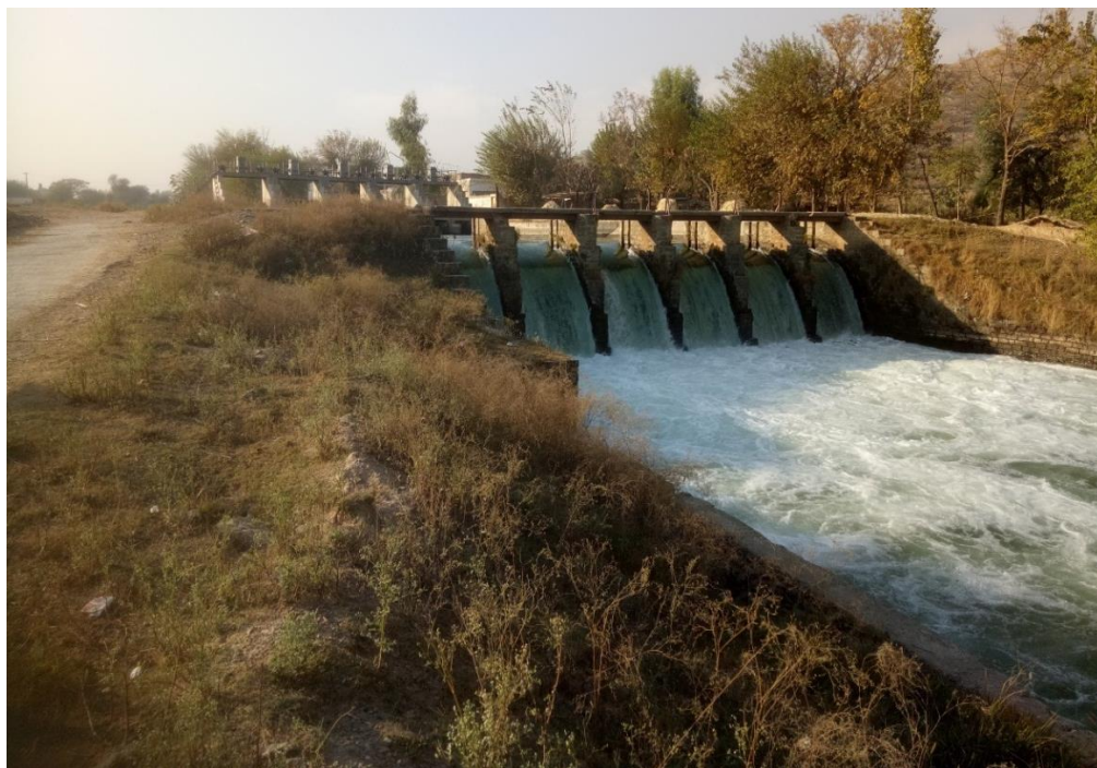
Annexure- II Fig: 0-1: The potential location of Machai canal available for submersible turbine project
