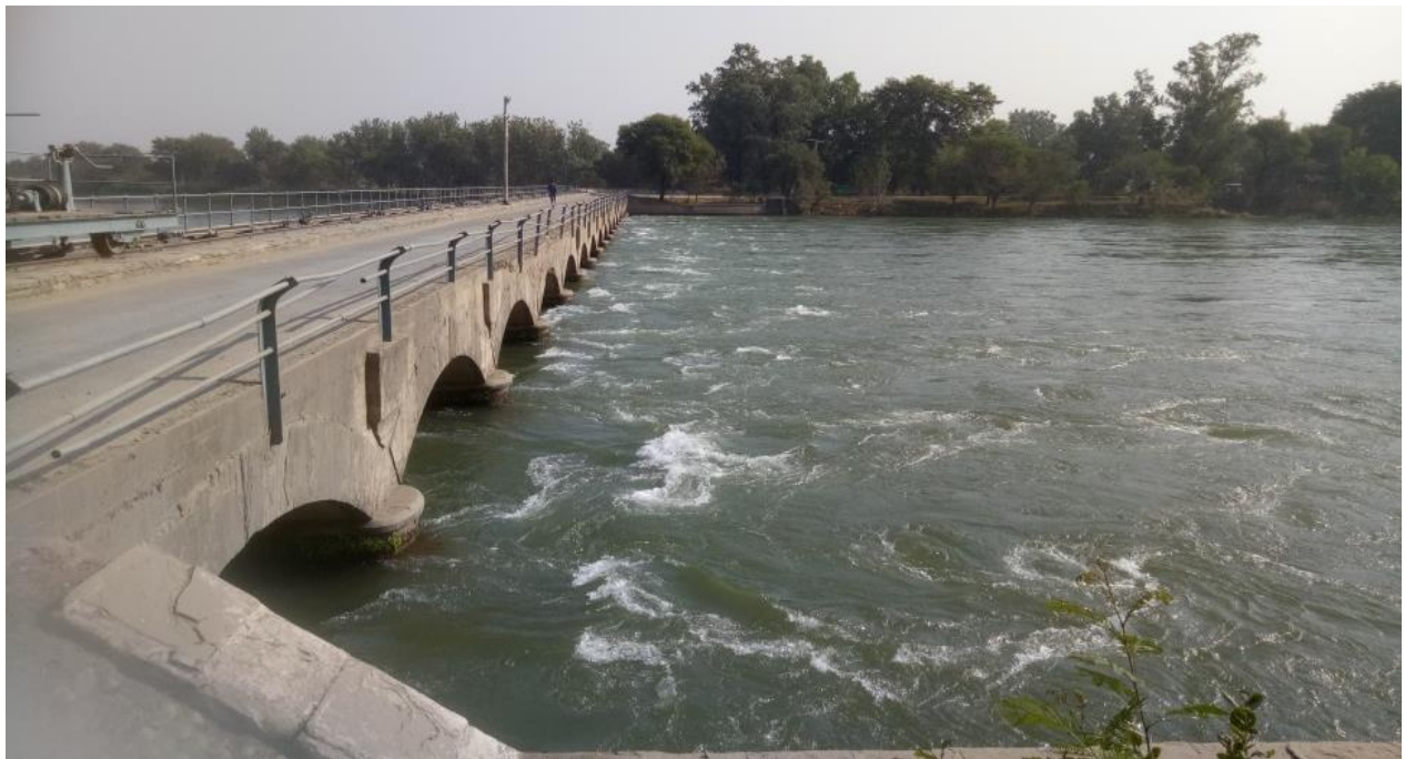
Annexure –III Fig: 0-2: Exact location for the installation, 2nd option at the exit of 2nd channel under the bridge.
