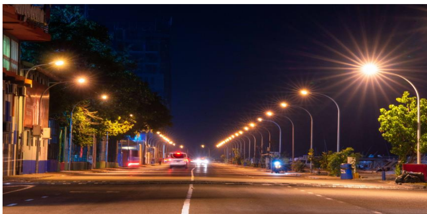
Figure- 15: Street Lighting of Male city of Maldives
