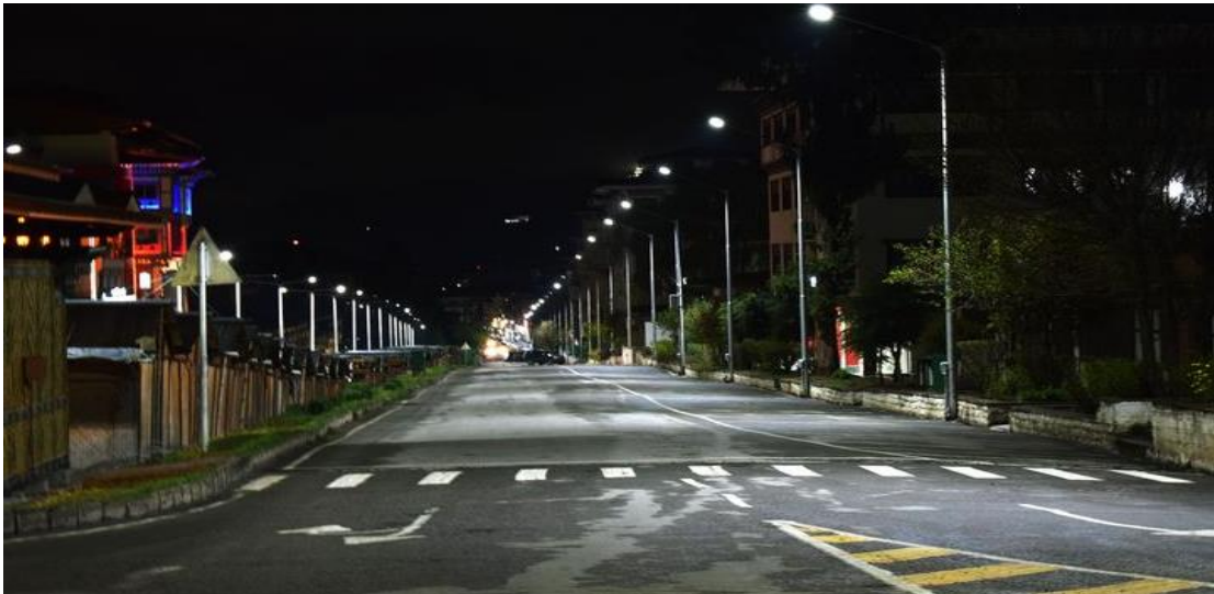
Figure- 13: Street Lighting of Bhutan roads
