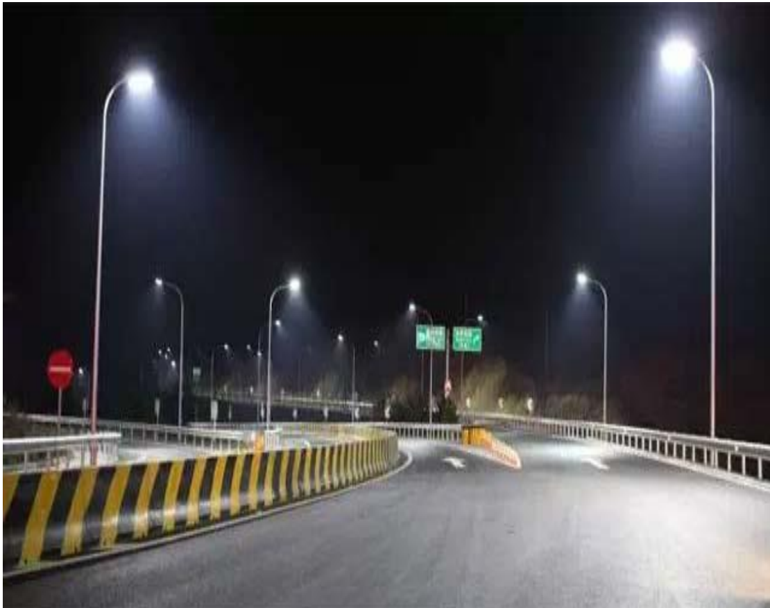
Figure- 26: Road Lighting Hyderabad City 69
