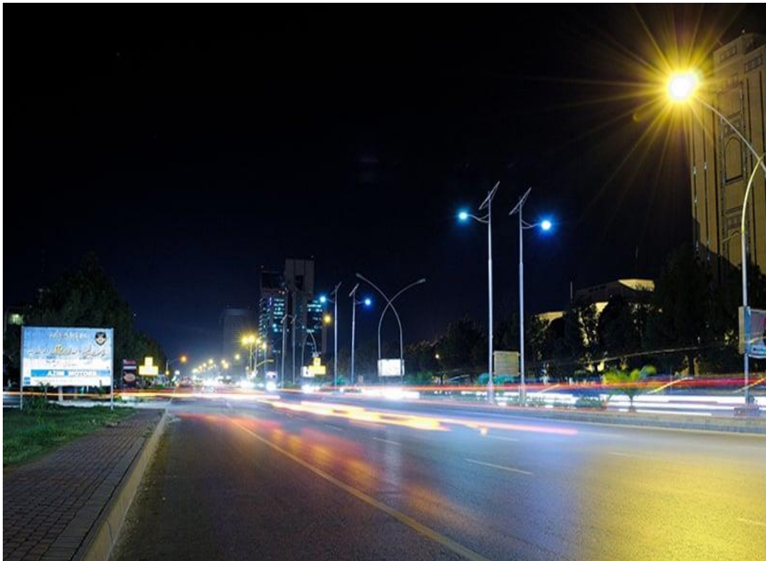
Figure- 29: Road Lighting of Islamabad City
