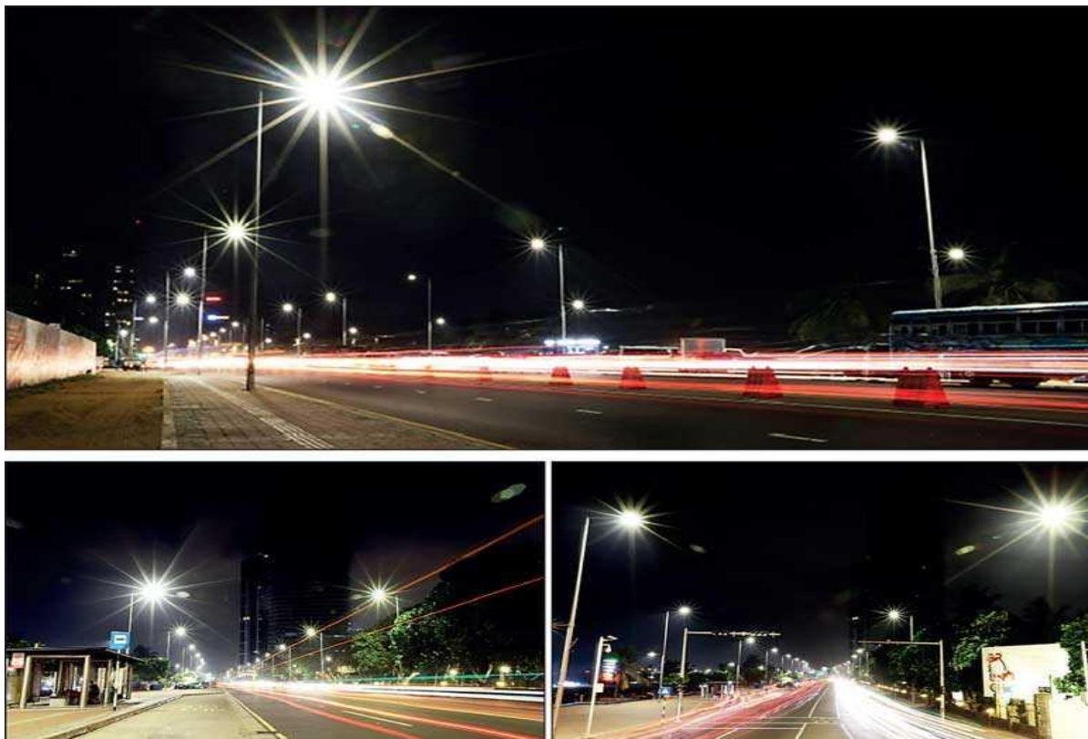
Figure- 18: Road Lighting Galle Road in Colombo City of Sri Lanka 20
