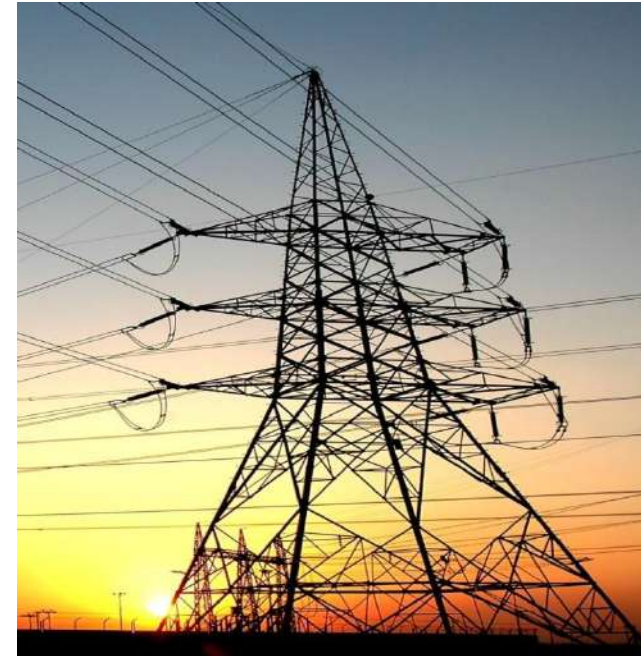
JUMPER SUSPENSION STRING
